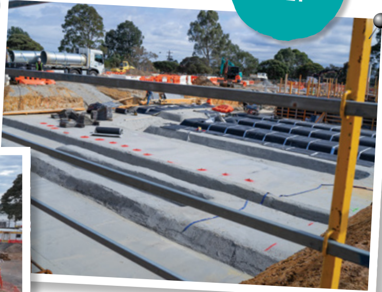
Image above: Concrete ridges indicate where heated coils will be located. Images left and below: Excavators prepare the hole for the 50-metre pool.
