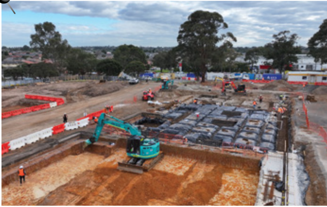
Image above: Concrete ridges indicate where heated coils will be located. Images left and below: Excavators prepare the hole for the 50-metre pool.
