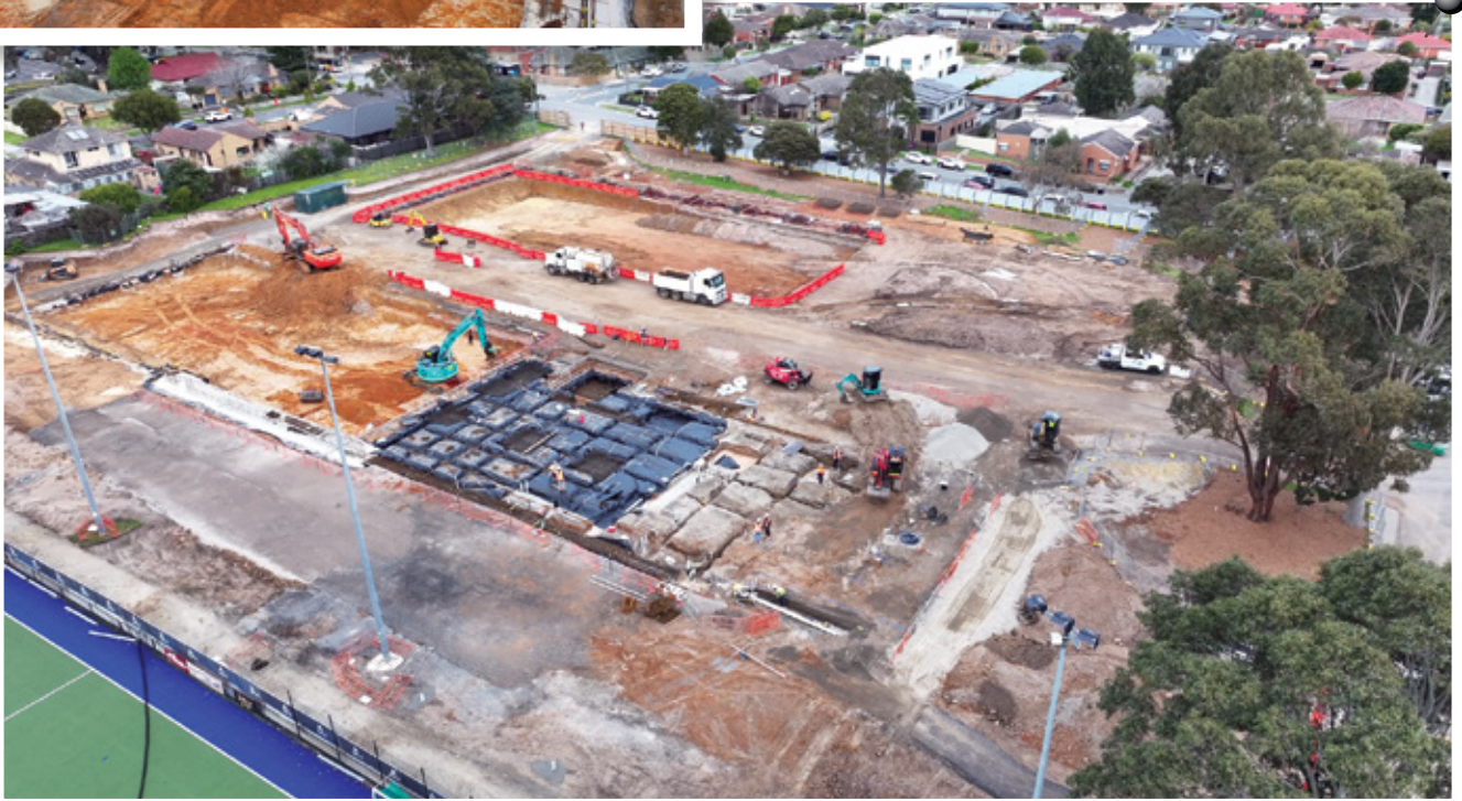
Image above: Concrete ridges indicate where heated coils will be located. Images left and below: Excavators prepare the hole for the 50-metre pool.
