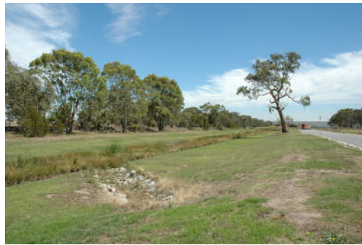
Figure 9 Example of treatment of watercourse within industrial estate.
