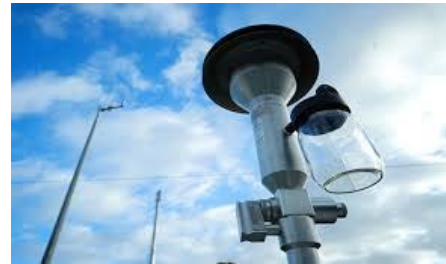
Figure EP – 2.3b Air Monitoring Station
