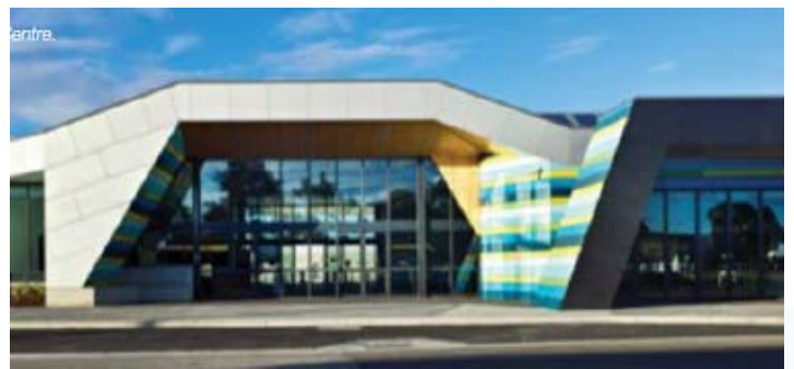
The Noble Park Aquatic Centre includes a 700,000-litre rainwater tank and use of grey water.
