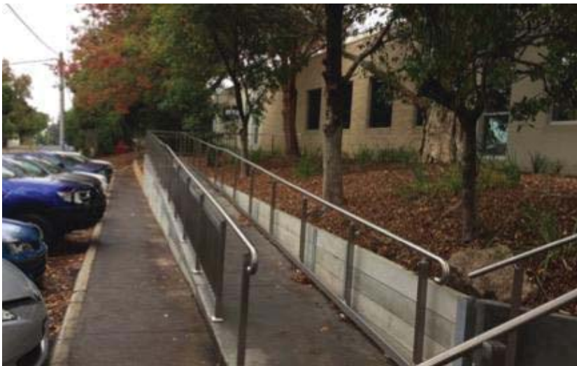
Image 13: Access Ramps and Walkways
