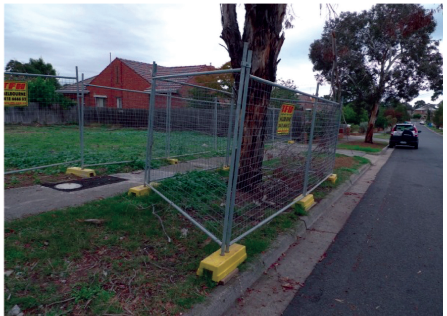
Figure 2: Photograph above left - example of signage for TPZ. Photograph above right - example of appropriate TPZ fencing around a street tree.
