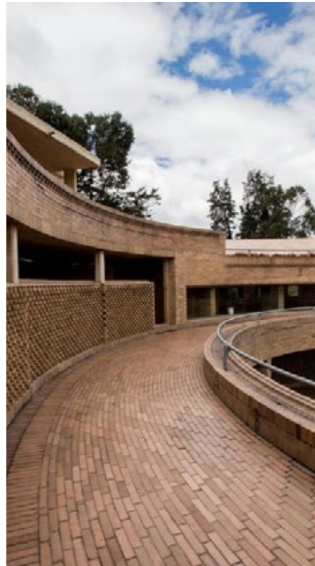
Radial red bricks create a smooth winding path
