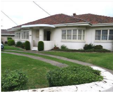
Figure 1: House from north (2021)
