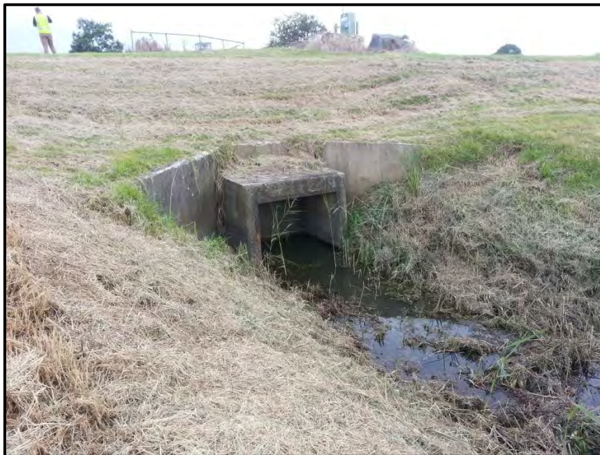
Figure 15 – Downstream outlet of the MW syphon under Dandenong Creek
