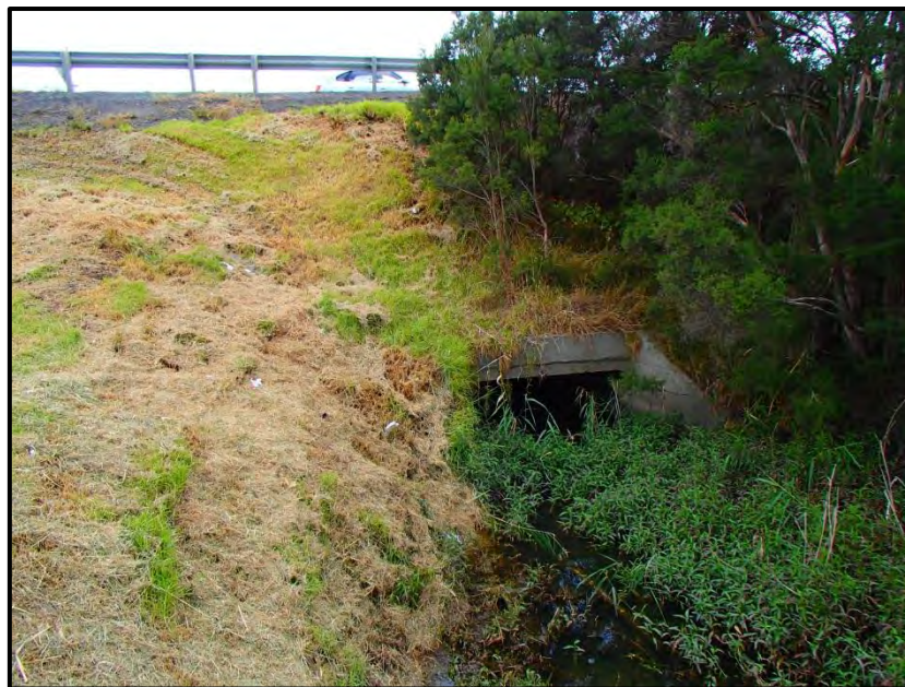
Figure 5 – Culvert under Perry Road (downstream of syphon)
