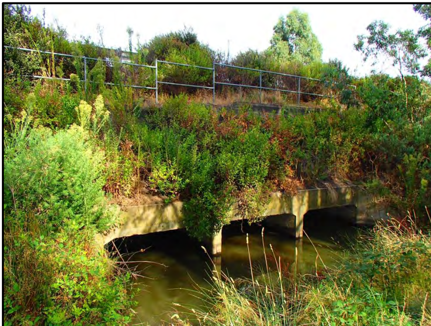
Figure 3 – Existing culverts under Perry Road at southwest corner of the site
