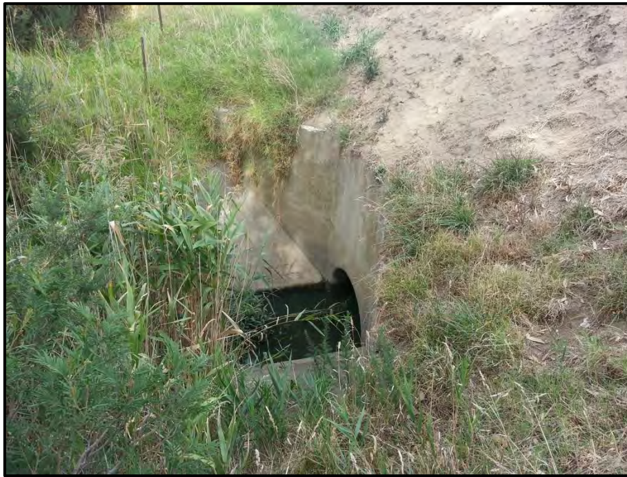
Figure 14 – Upstream inlet of the MW syphon under Dandenong Creek
